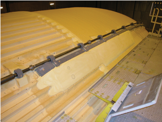
Shown here is the liquid oxygen PAL ramp
