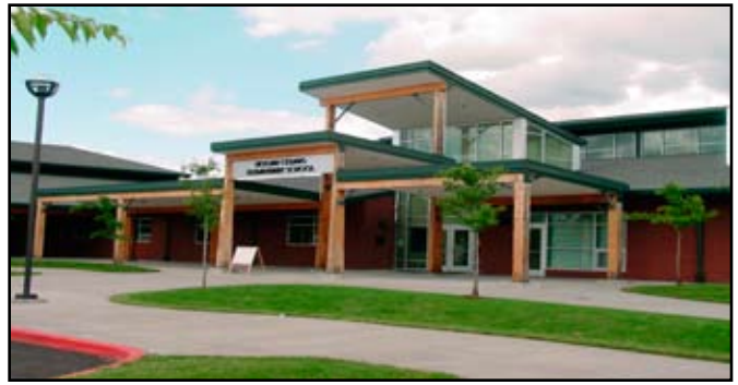
Recently constructed Hogan Cedars Elementary has clerestory windows that provide sufficient natural light and reduce electricity use.
