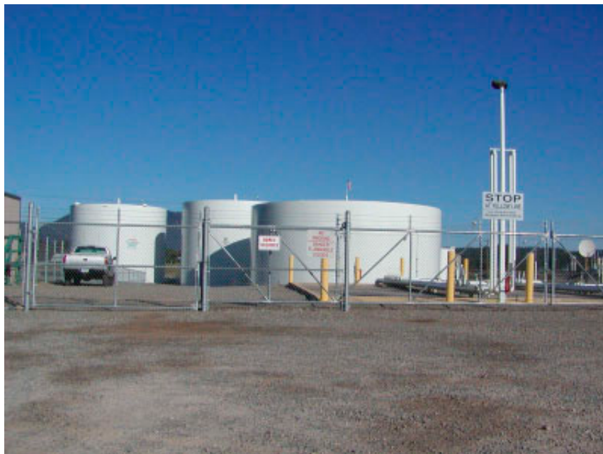
Rail Terminal in Montana
