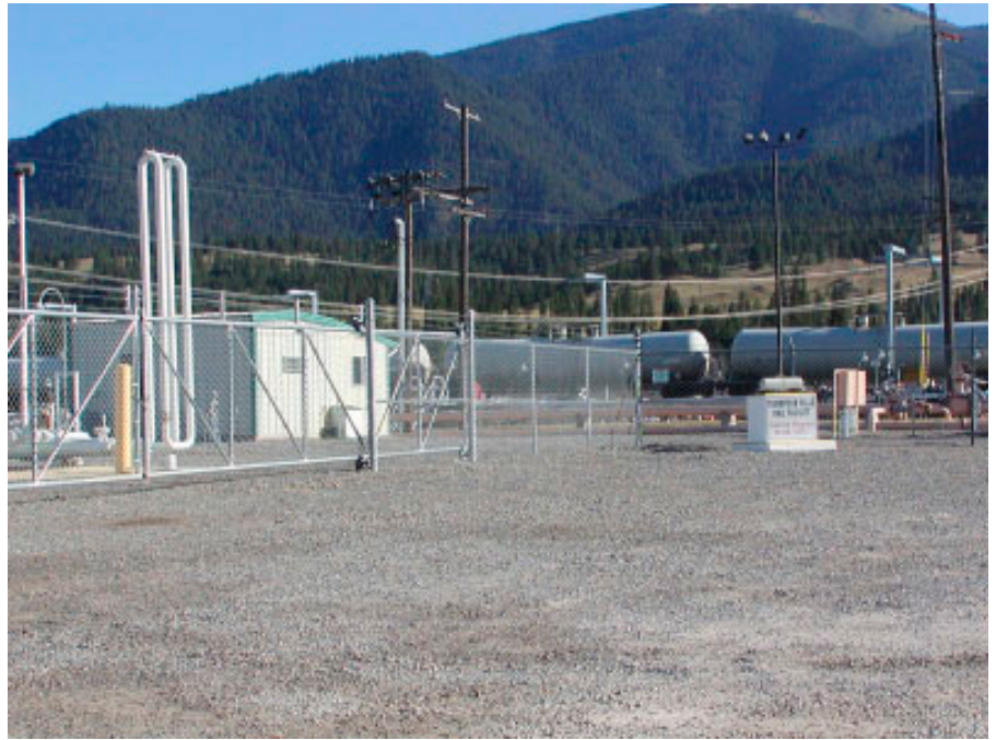
Thompson Falls Rail Facility
