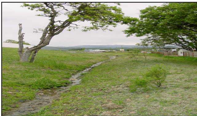
The bioswale behind the school effectively filters rain runoff before it enters the city storm system.
