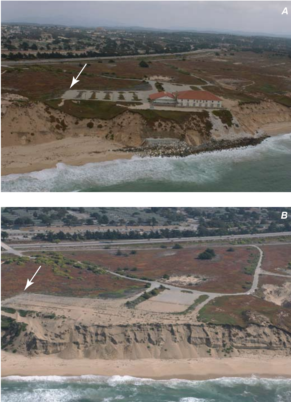
Figure 24. Stillwell Hall, a soldier's club on the Fort Ord military base, was threatened by rapid erosion of the bluffs for years before being removed in 2004: A) Stillwell Hall in 2002 with riprap revetment along base of bluff. The arrow points to a corner of the parking lot for reference; and B) the former site of the hall in 2005. The arrow points to the same location as in A. The amount of retreat measured over 70 years in this area was just over 116 m. (Photos copyright (c) 2002-2007 Kenneth & Gabrielle Adelman, California Coastal Records Project, www.californiacoastline.org ).
