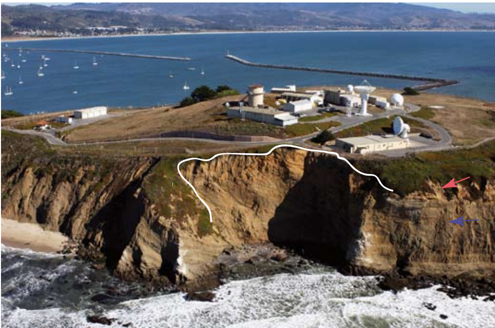
Figure 21. The headland at Pillar Point is composed of sands and gravels (red arrow) overlying mudstone (blue arrow). The poorly lithified sand and gravel are eroding rapidly, and as a result the cliff has retreated 210 m over a 70-year period. The white line outlines the head scarp of the actively eroding portion of the cliff. (Photo copyright (c) 2002-2007 Kenneth & Gabrielle Adelman, California Coastal Records Project, www.californiacoastline.org ).
