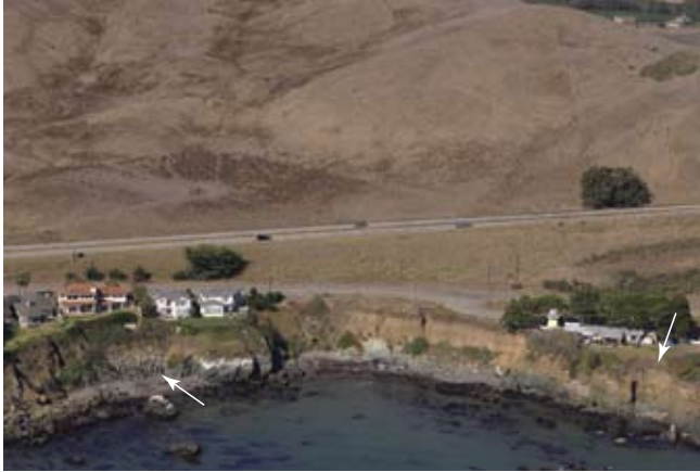
Figure 28. Retreat of the low coastal cliff threatens these homes near Cayucos Beach (see Figure 10B for reference). The cliff retreat at this location was 33 m over the 70-year time period of this study. The left arrow points to riprap at the base of the bluff, and the right arrow points to a portion of actively eroding bluff. (Photo copyright (c) 2002-2007 Kenneth & Gabrielle Adelman, California Coastal Records Project, www.californiacoastline.org ).
