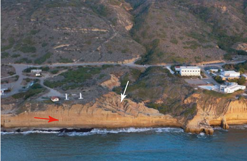
Figure 40. The maximum cliff retreat (-100 m) and the highest retreat rate (-1.6 m/yr) in the San Diego region were measured at the site of the Point Loma Nazarine College. Along this section of coast, the rocks at the cliff base are more resistant to wave attack (red arrow) and the unlithified upper cliff materials are rapidly eroding through processes of gully and rill formation (whiter arrow). (Photo copyright (c) 2002-2007 Kenneth & Gabrielle Adelman, California Coastal Records Project, www.californiacoastline.org ).
