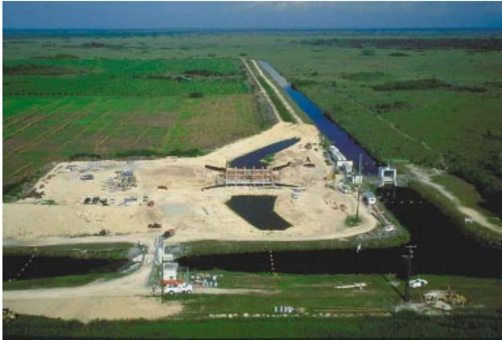
Pumping facility under construction adjacent to Everglades National Park
