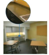
EPA installed two pantries on every floor using **sustainable materials** and finishes such as recycled aluminum in counter tops, metal laminate cabinetry, linoleum flooring, and rubber bases. The pantries are stacked from floor to floor so they can easily direct exhaust to the outside, maintaining IAQ. ENERGY STAR refrigerators and microwaves are located in the central pantries for **energy efficiency**.
