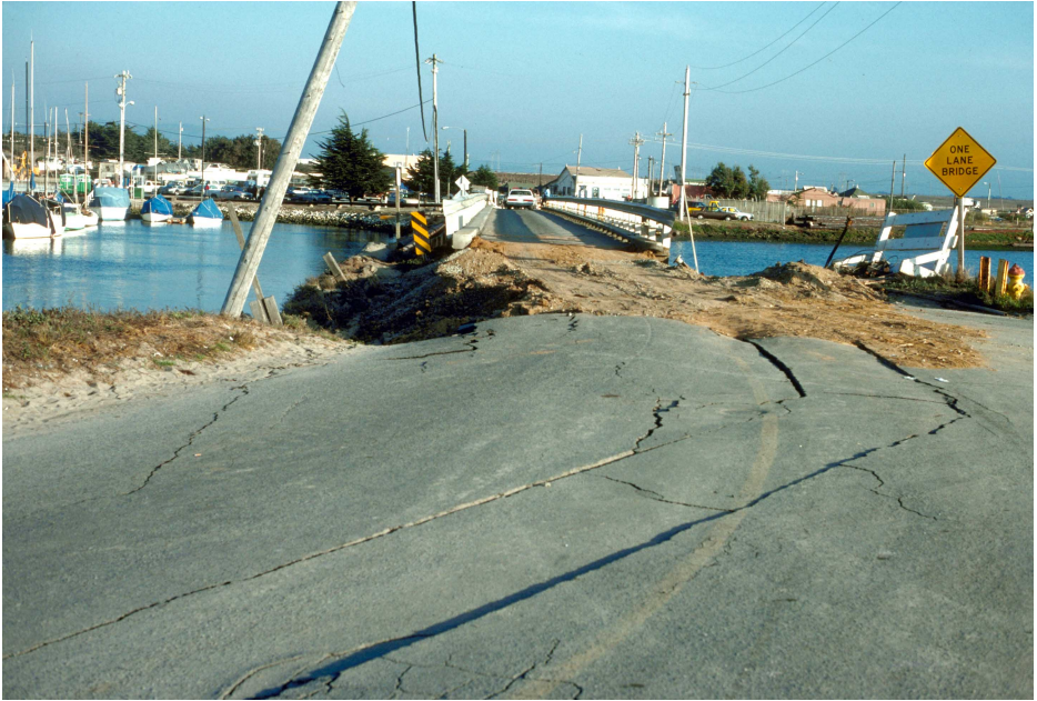
101. Ground cracking and differential settlement due to liquefaction of beach and Salinas River deposits damaged approach and abutment of bridge linking Moss Landing spit to the mainland, near Moss Landing Marine Laboratory. [J.C. Tinsley, U.S. Geological Survey]
