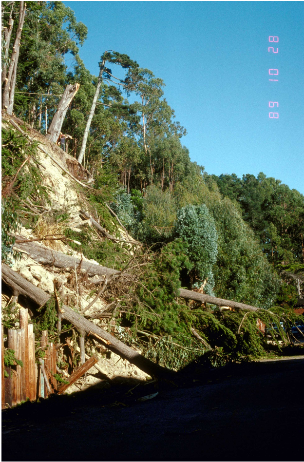
83. Landslide-displaced trees reflect earthquake-triggered slope failure along coastal bluff, New Brighton Beach area, Santa Cruz County. [J.C. Tinsley, U.S. Geological Survey]
