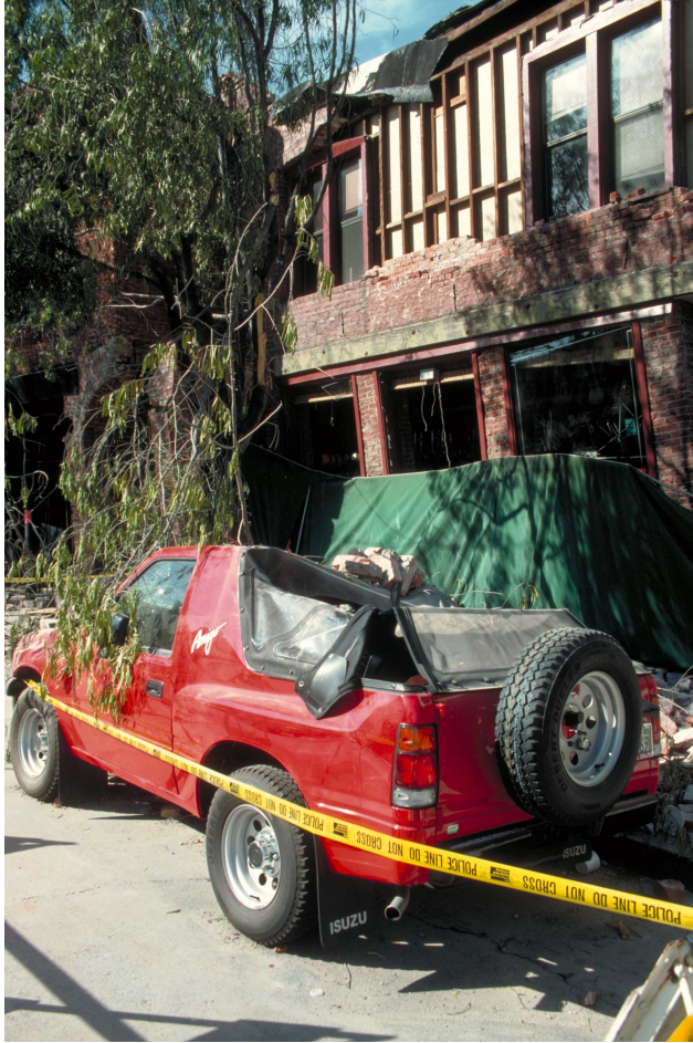
51. Vehicle crushed by collapse of unreinforced-brick masonry. [C.E. Meyer, U.S. Geological Survey]
