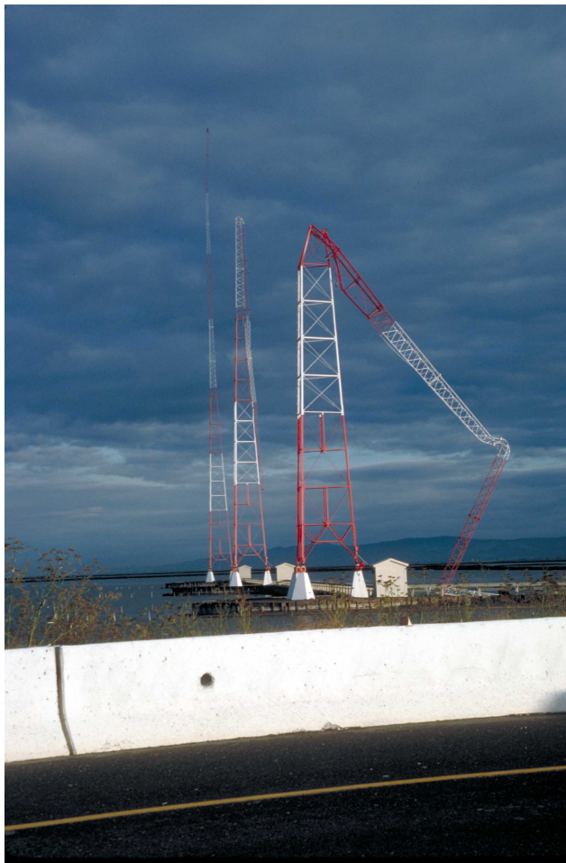
37. KGO radio transmission towers, built on bay mud in a salt-evaporation pond used by the Leslie Salt Company. Note progressively less damage to towers away from viewer. [H.G. Wilshire, U.S. Geological Survey]
