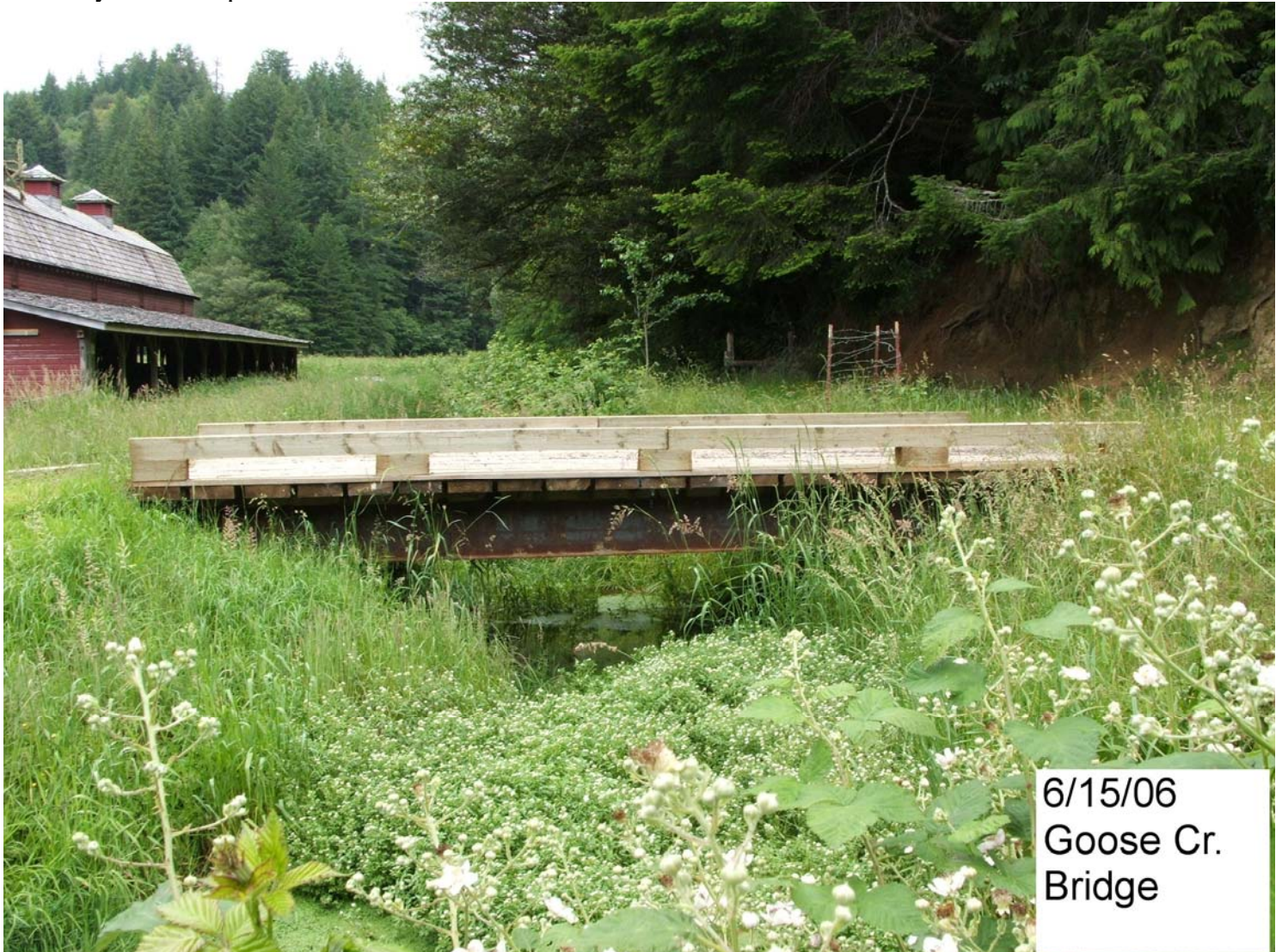
Photo 1. Summer monitoring photo of Goose Creek Bridge site.
