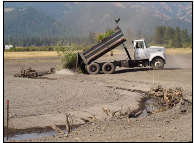
Dump truck hauling and stockpiling plant materials at selected locations along End Creek restoration channel. September 2006.
