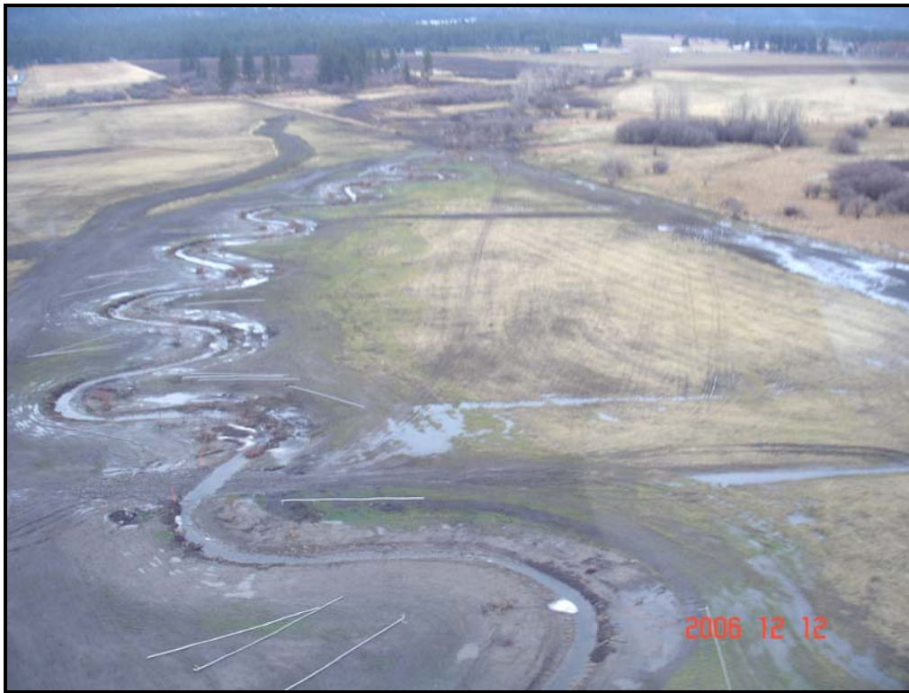
Upstream view of upper End Creek restoration channel. December 2006
