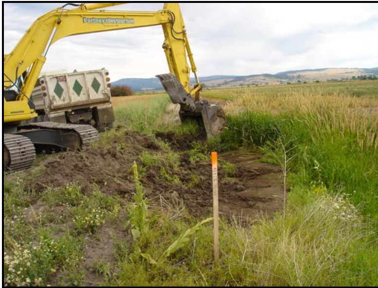
Initiation of End Creek restoration channel construction. July 2006
