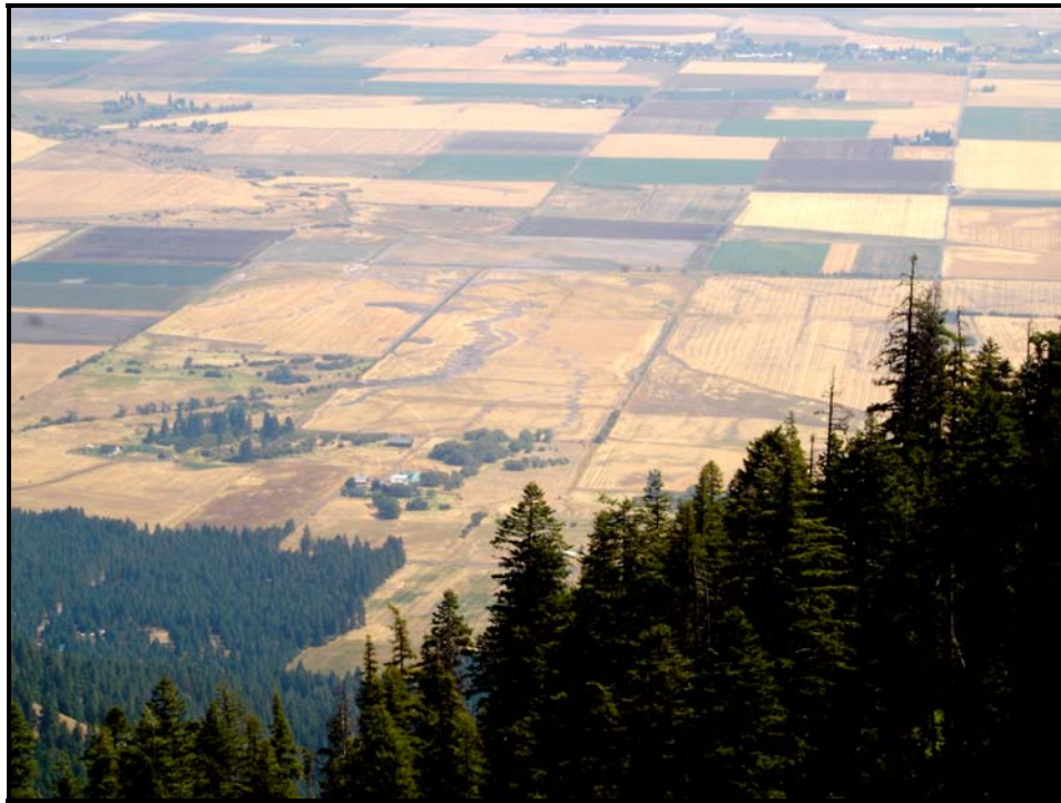
End Creek Restoration Project Complex. Summer 2006 Construction viewing northeast from Grandview Campground atop Mount Emily
