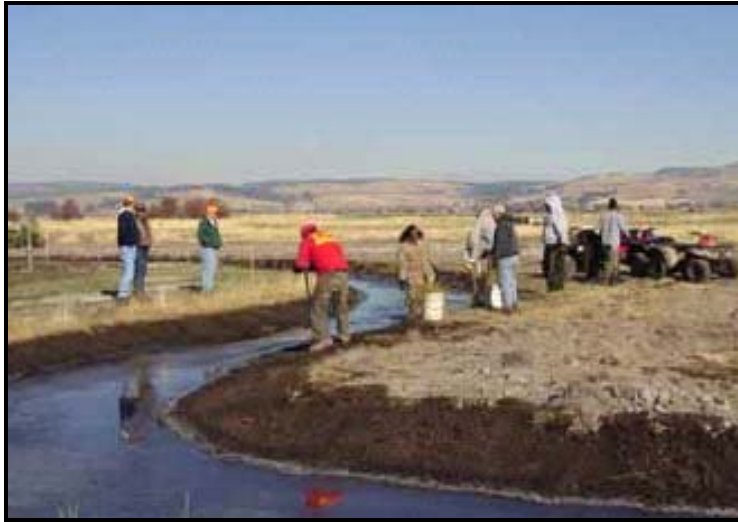
CTUIR habitat crew installing sedge/rush plugs along South Fork Willow Creek. October 2006
