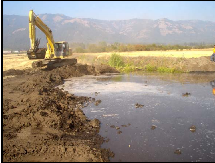
Floodplain pond construction. August 2006.
