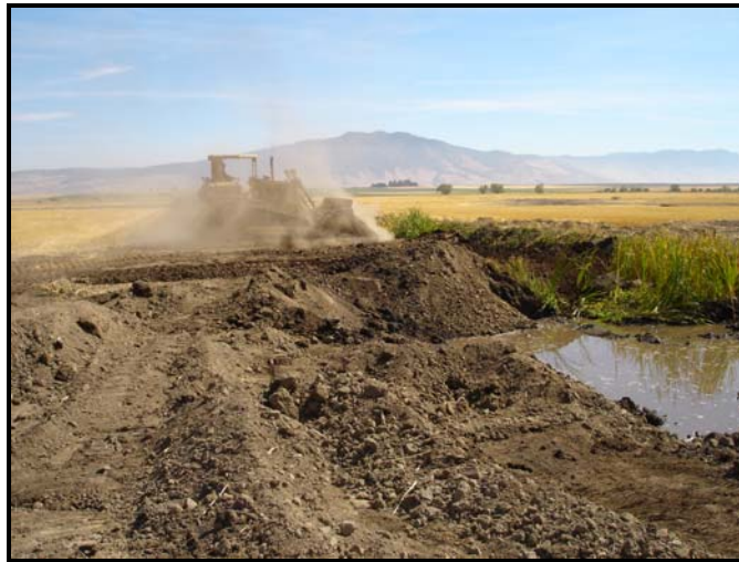
Reclamation of channelized End Creek following activation of restoration channel. August 2006.
