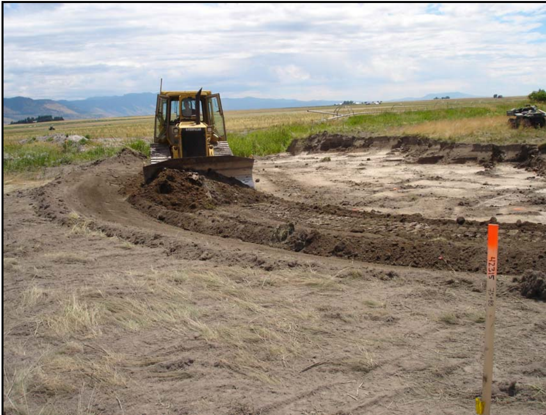
Initiation of channel construction on lower End Creek. December 2006
