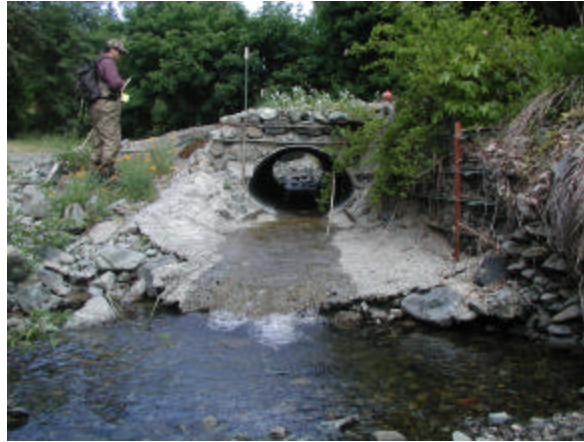
Figure 8. Private drive culvert (H15), Humbug Cr.
