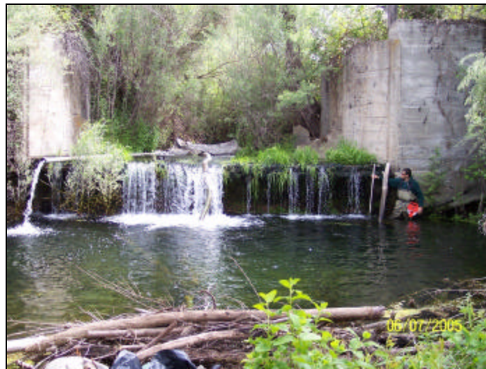
Figure 5. Cement barrier below confluence of Bishop Creek.
