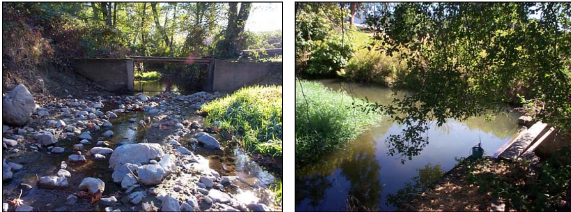
Figure 3.1: Jones Creek Irrigation Diversion
