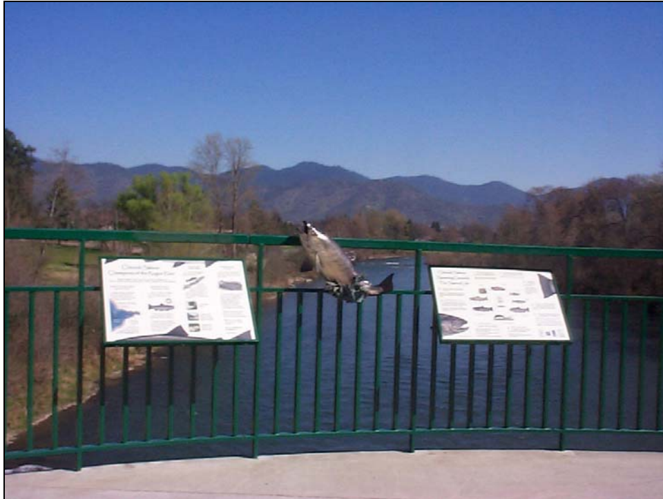
All Sports Park Bridge in Grants Pass
