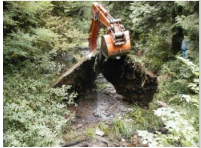
One of the Hogans Cedar Dams on Johnson Creek being removed.
