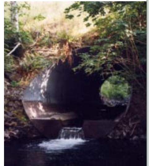
Culvert blocking fish passage on Deep Creek prior to installation of a bridge.
