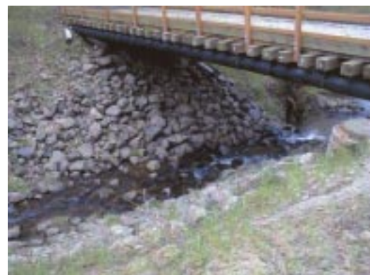
Boxler Creek now provides fish passage after installation of a bridge.
