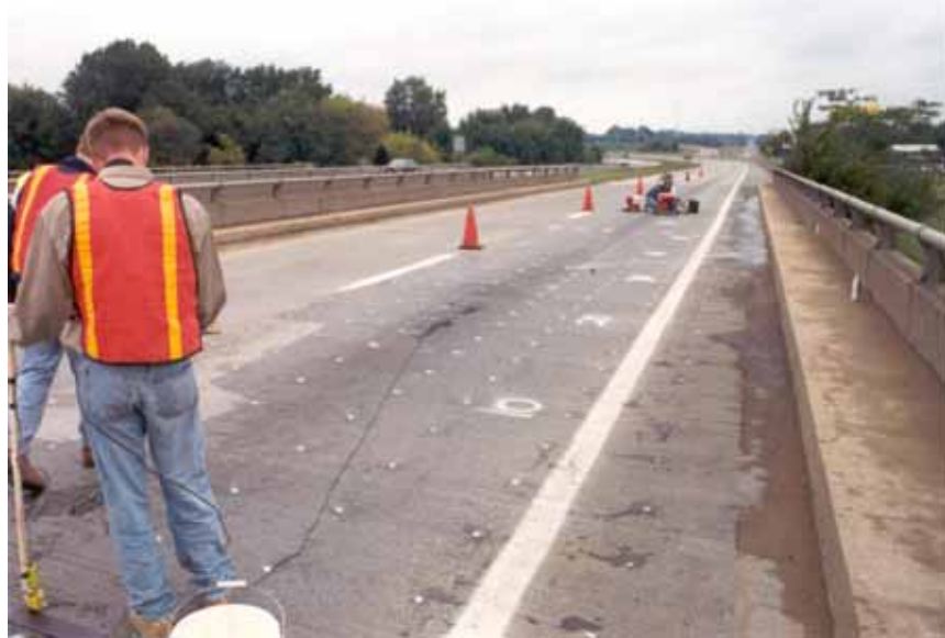
Figure 24. Photograph of southbound test section of U.S. 41 (silica fume concrete overlay).
