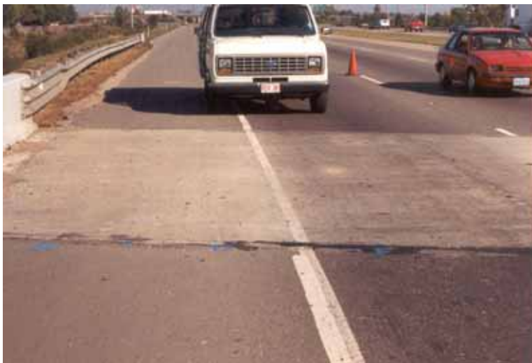
Figure 3. Photograph showing test section on I-270 southbound (1995).
