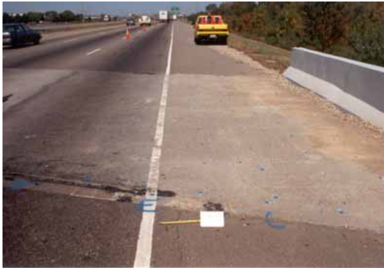
Figure 2. Photograph showing test section on I-270 northbound (1995).
