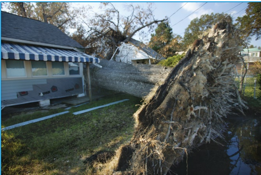
Hurricane Isabel wind damage, Colonial Beach, VA September 30, 2003/ Photo by Andrea Booher/FEMA
