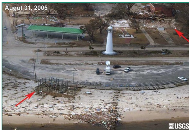
After Hurricane Katrina August 31, 2005— Biloxi, MS/USGS
