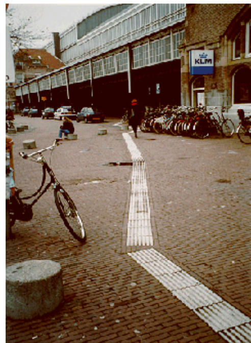
Figure 11. Guidance strip for visually handicapped.
