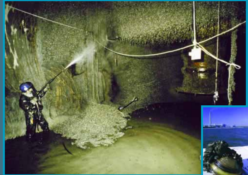
Workers remove zebra mussels from a water intake pipe at DTE Energy's Monroe Power Plant
