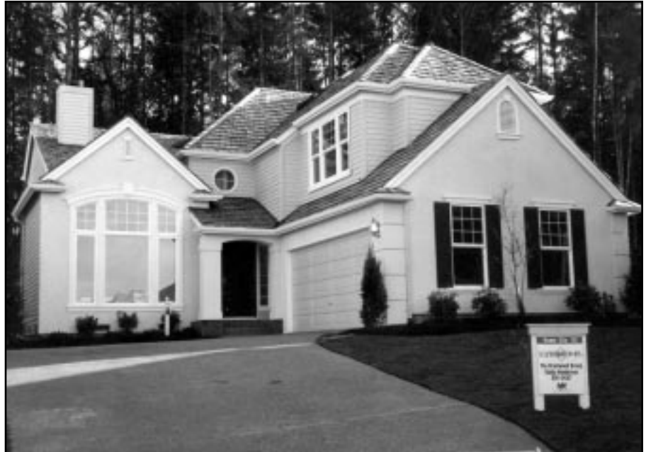
A new Lozier home in the Klahanie development in Issaquah. Job-site recycling on the entire 60-home project saved nearly $15,000.
