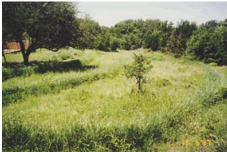
Figure 5 This sloped bioretention facility was a more cost-effective design for an Austin, Texas subdivision than a conventional pond. Photo courtesy of Murphee Engineering.
