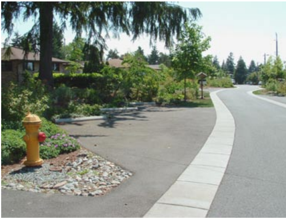
Figure 3.9 Pullout parking adjacent to a 14-foot residential access road, Seattle.
