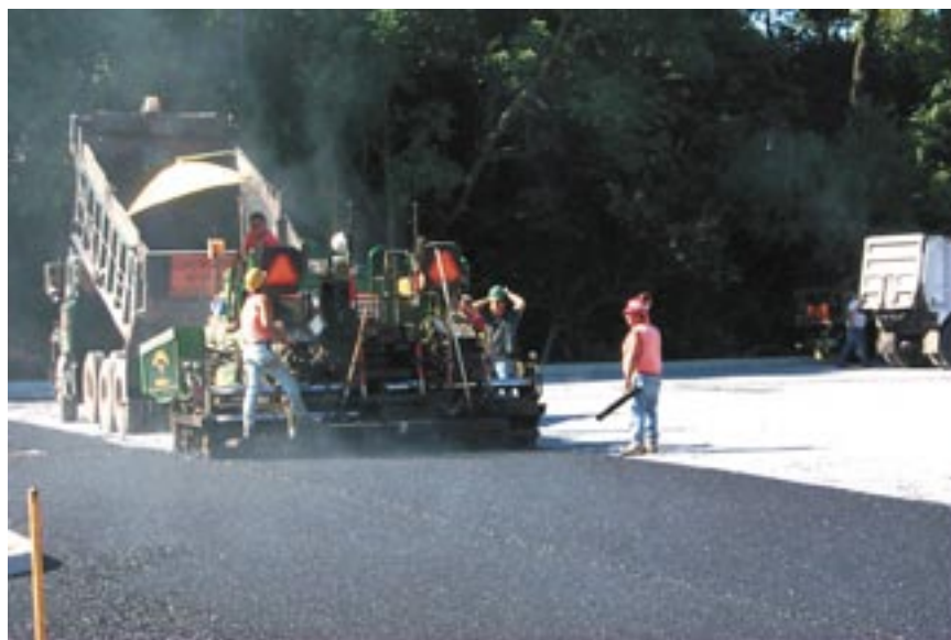
Figure 1 Parking installation, Courtesy of Cahill Associates
