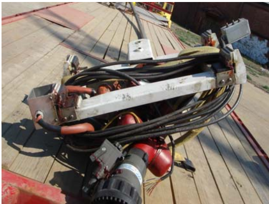
Photo 4 – Monitor and pipe that “launched”
