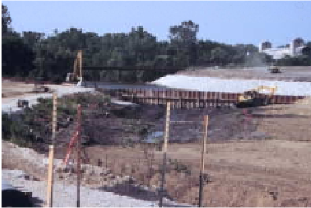
Ottawa River cleanup site, completed under a unique public/private partnership.
