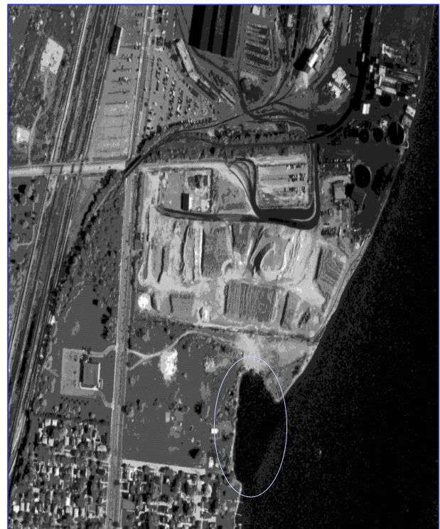
Site of planned cleanup in the Black Lagoon on the Detroit River where maximum contaminant concentrations include mercury (7.8 ppm) and oil and grease (20,000 ppm).
