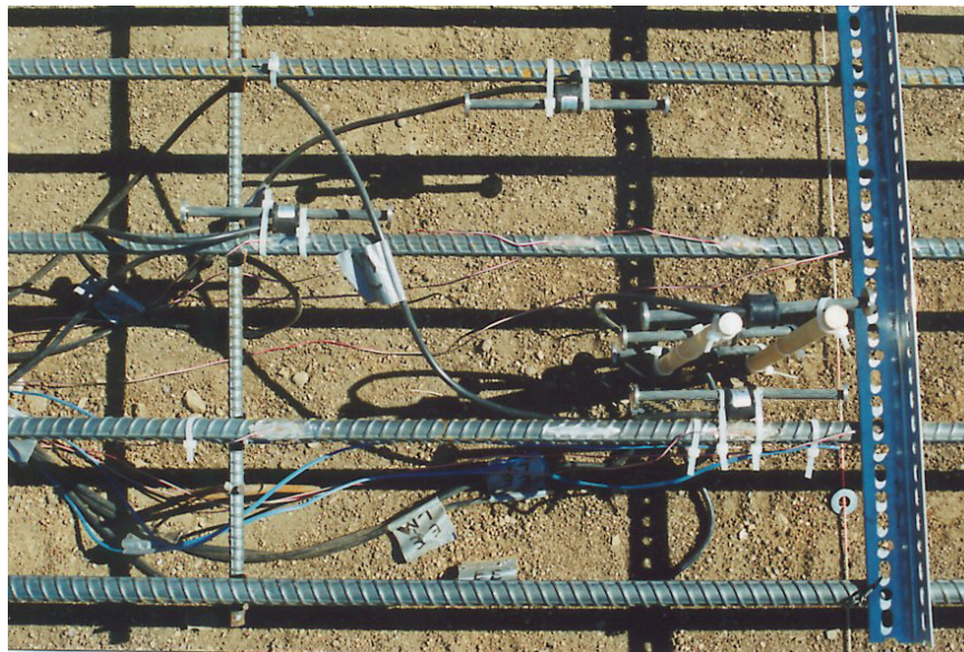
Figure 92. Strain gages in PCC and on reinforcing steel.
