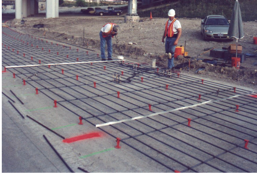
Figure 87. Instrumented section delineated by crack inducers.
