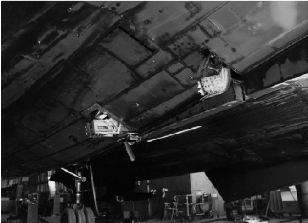
During a low-speed functional check flight of the YF-12A with the Coldwall experiment attached, the aircraft's ventral fin tore off. Although the right wing was damaged, causing a fuel leak, the pilot, Don Mallick, landed safely at Edwards. (NASA photo E75-28266)
