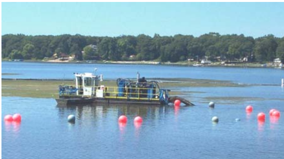
Suction dredge removing Tannery Bay sediments
