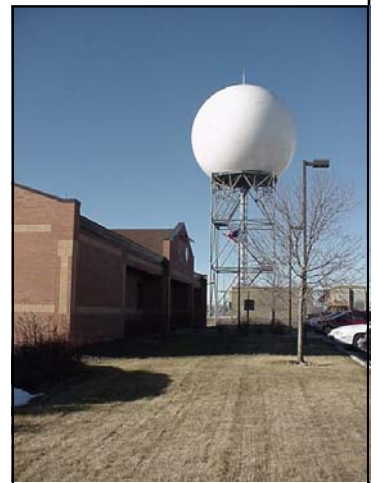
The radar located next to the Cheyenne Weather Forecast Office
