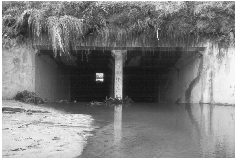
Figure VI-21--Double Barrel Box Culvert
