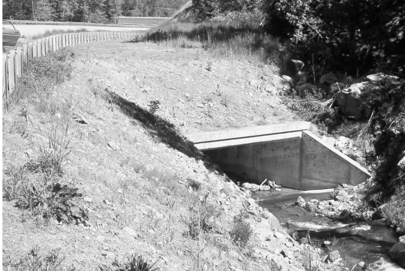
Figure VI-20--Fill Warped to Avoid Inlet Skew
