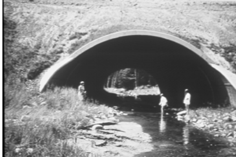
Figure I-2--Long Span Culvert
