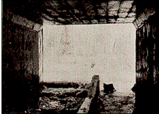
Figure VI-7--Fish Baffles in Culvert
