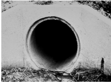
Figure I-1--Typical Concrete Pipe Culvert
