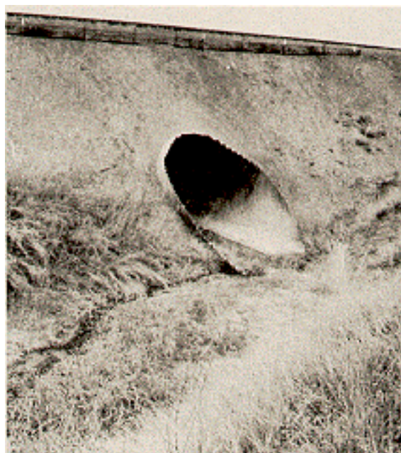
Figure VI-33--Unanchored Mitered End
