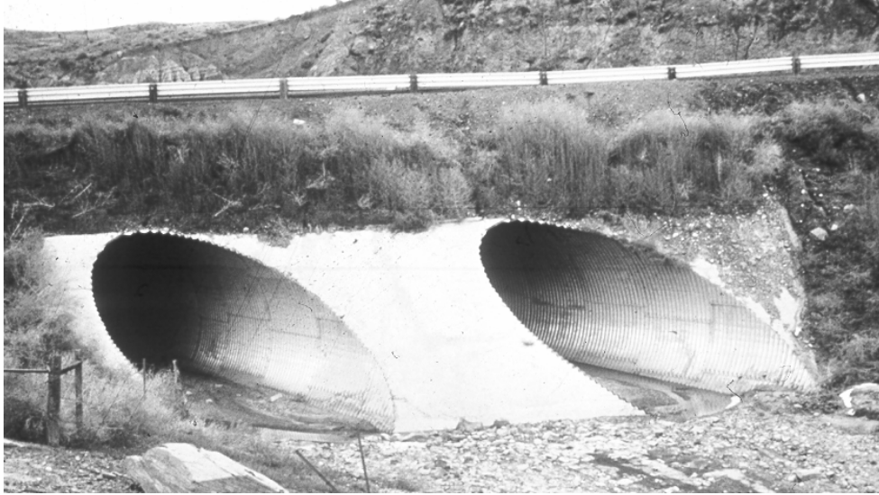
Figure VI-34--Slope Paving Around a Mitered Inlet
