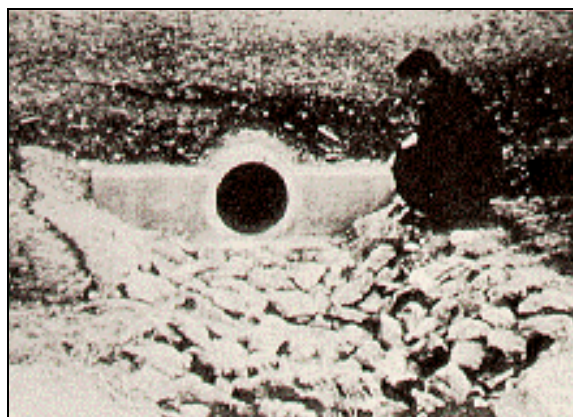
Figure VI-14--Riprap Protection at Culvert Outlet
