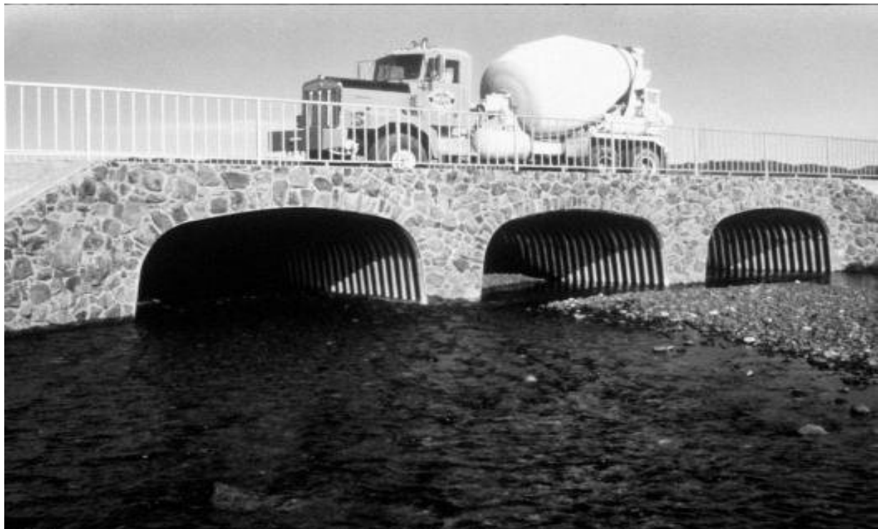
Figure VI-24--Corrugated Metal Box Culvert (Contech)
