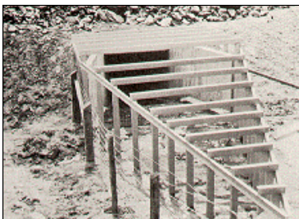
Figure VI-16--Debris Deflector
