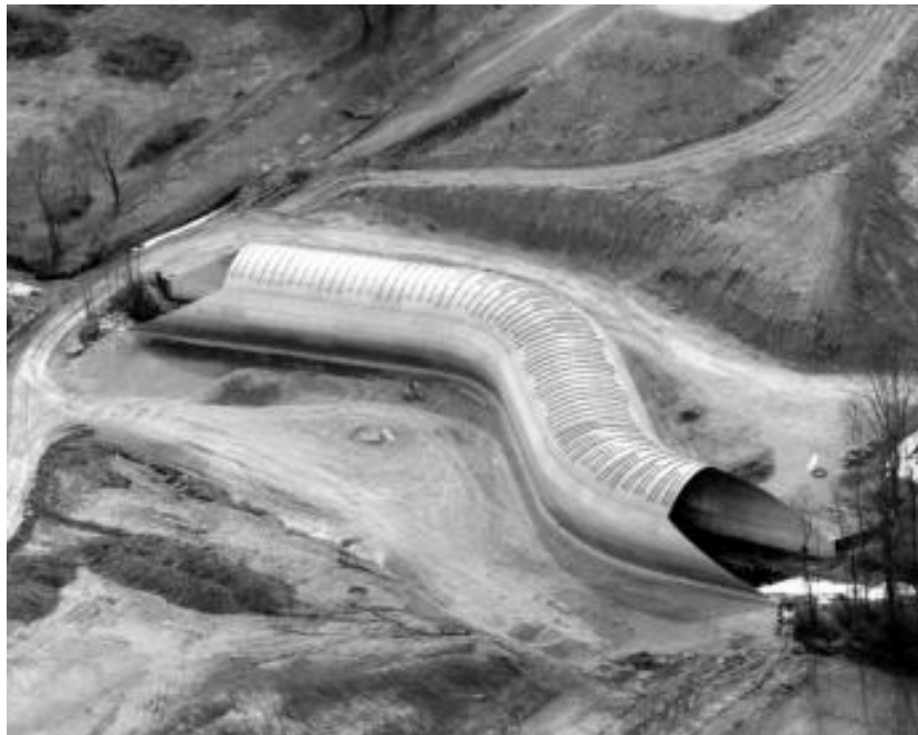
Figure VI-4--Culvert with a Horizontal Bend (Contech)
