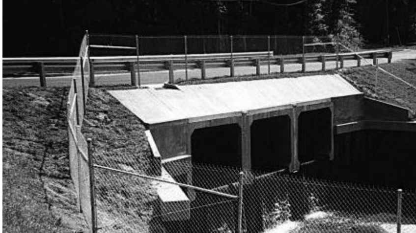
Figure VI-28--Guardrail Adjacent to Culvert Headwall (American Concrete Pipe Association)
