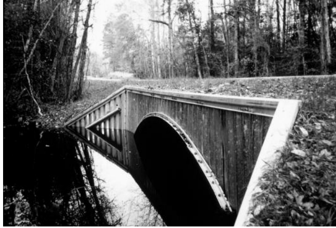
Figure VI-10--Culvert with Metal Headwall and Wingwalls (Contech)
