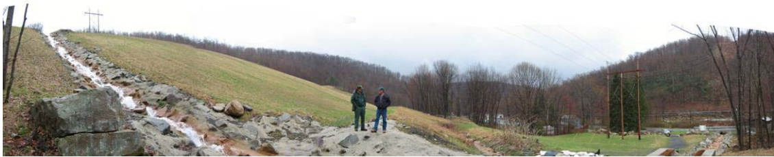
Shallmar Title IV Reclamation Project
