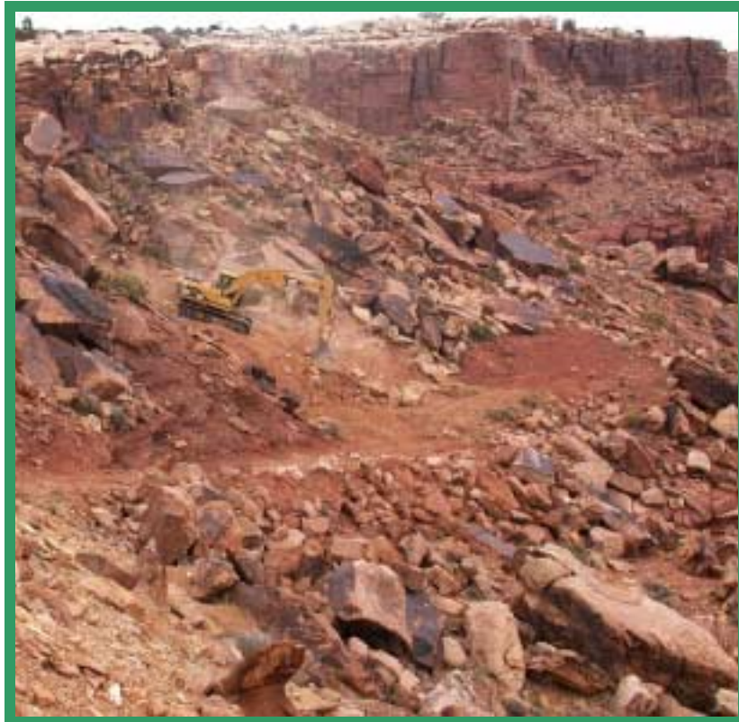
Shima Mine: Excavator performing backfill closure of uranium portal.
