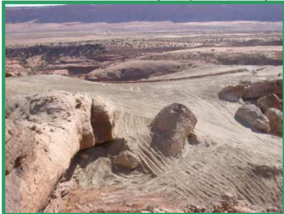
Cove-3 Reclamation Project after reclamation. Prior to reclamation this was a very steep and treacherous area.
