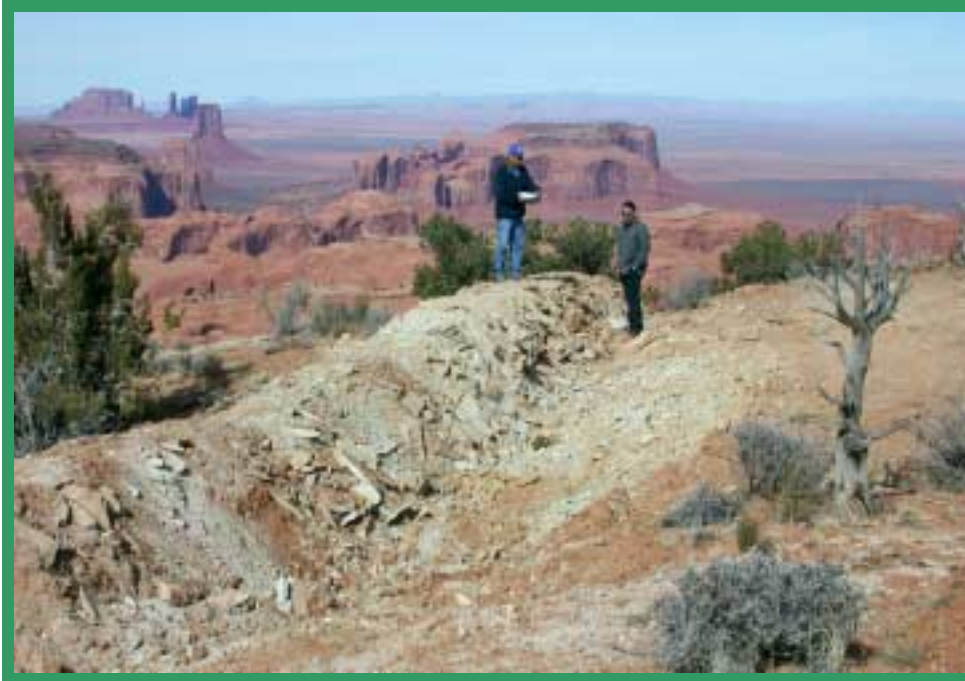
Monument Valley-4 Project: Reclamation berm to control drainage leaving reclaimed area. Monument Valley Scenic Park is in the background which surrounds the project to the north.
