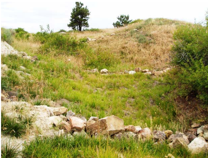
Luther 1 Mine photo July 2007 showing excellent utilization of rock check dams to control runoff
