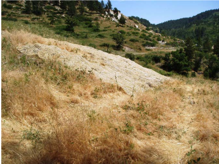
Larance Mine Maintenance photos July 2007 showing use of straw netting to repair erosion on reclaimed outslope and road cut
