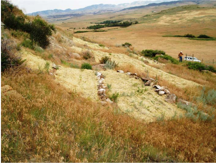
Matt Mine photos July 2007 showing excellent utilization of straw netting for erosion control and vegetation establishment
