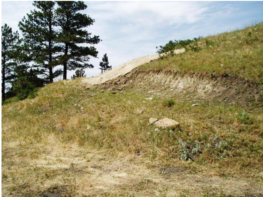
Larance Mine Maintenance photos July 2007 showing use of straw netting to repair erosion on reclaimed outslope and road cut
