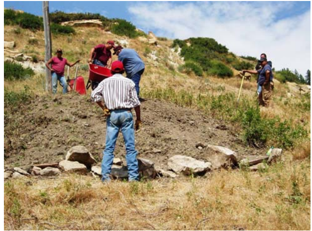
William T. Shaw Mine Maintenance photos July 2007 showing initial work to cover exposed coal and control erosion
