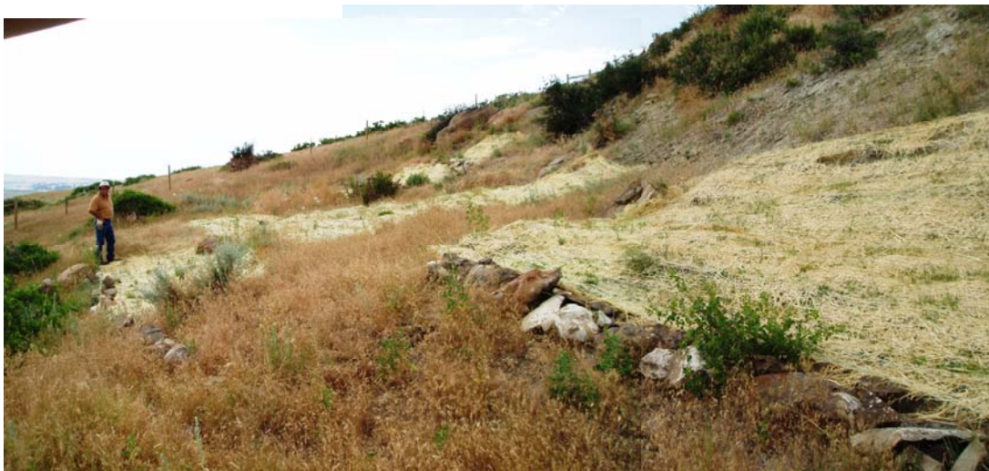
Matt Mine photos July 2007 showing excellent utilization of straw netting for erosion control and vegetation establishment
