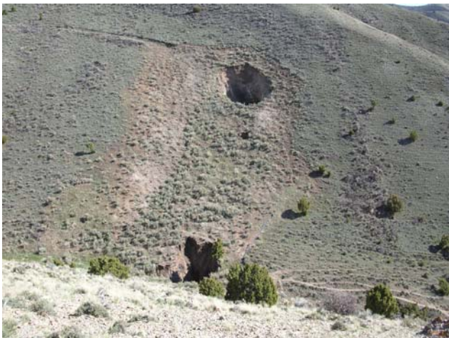
Photo 3. Reclaimed crown pillar line and new subsidence openings near former subsidence features E353, E352, and E350 of the Otto project. April 24, 2007.
