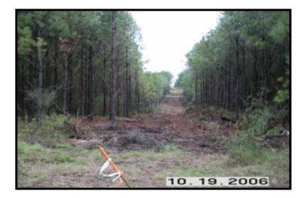
• Topsoil substitute has been scraped aside and used as fill. Material that was covered with the topsoil substitute has been exposed (See photograph below).
