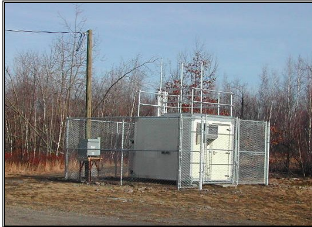
Centralia air-monitoring station
