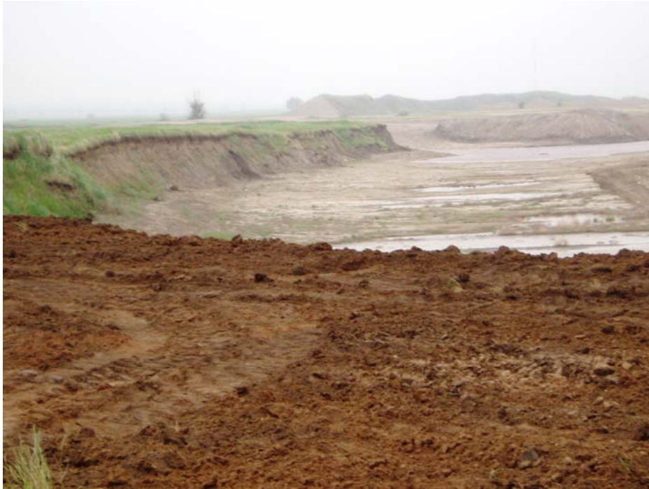
Columbus VIII Project (during reclamation) highwall elimination
