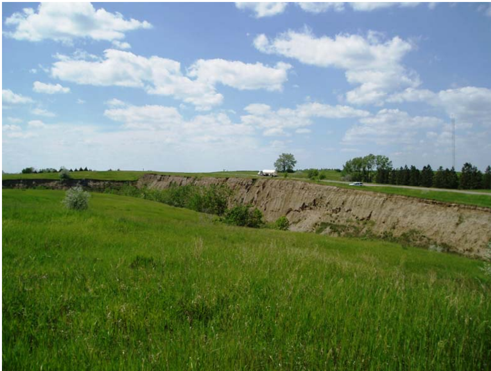
Highwall hazard adjacent to N.D. Highway 200 between Beulah and Hazen , North Dakota
