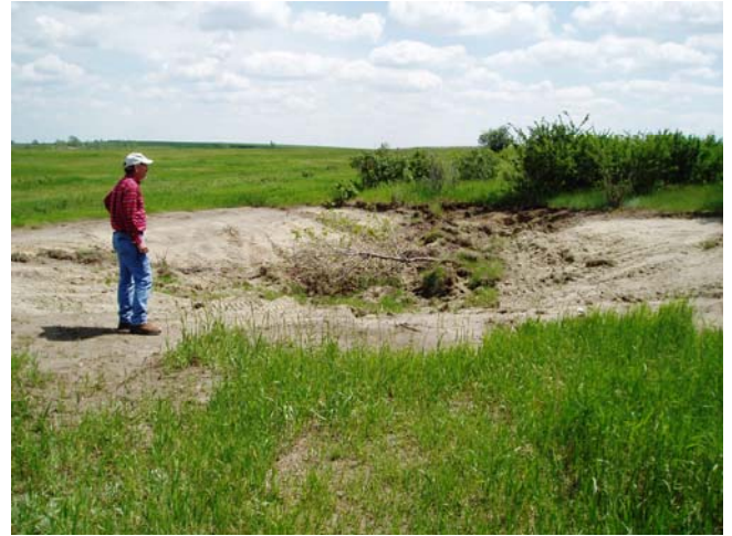
2006 Sinkhole Maintenance Project included elimination of sinkhole in left photo
