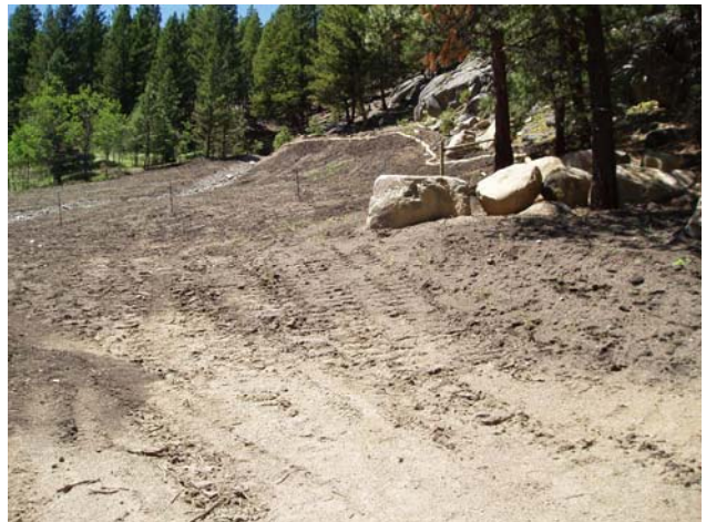
Big Chief Mine , photos above & below June 2007 (reclamation nearing completion) showing mine wastes piles removed, areas regraded, drainage channel reestablished
