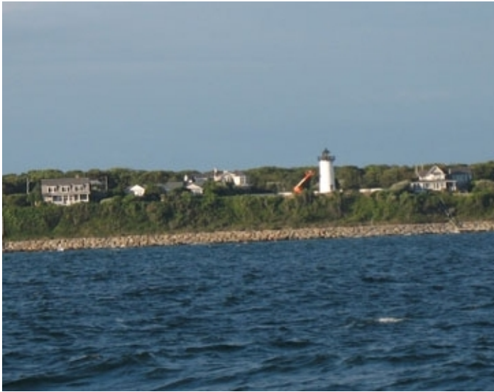
Martha's Vineyard Lighthouse being restored
