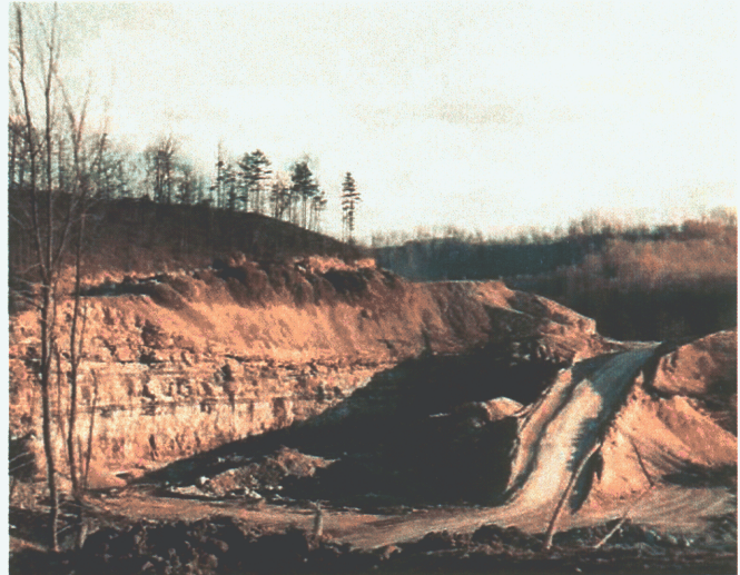
3b. Contouring overburden blasting in Perry County, Kentucky.
