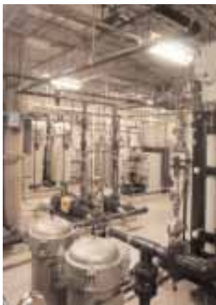
Source: The Austin Company, Designer-BUILDER
