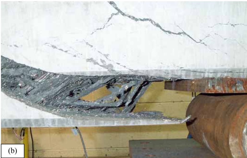
Figure 39. Photo. Failed Girder 24S (a) south elevation and (b) bottom flange near bearing.
