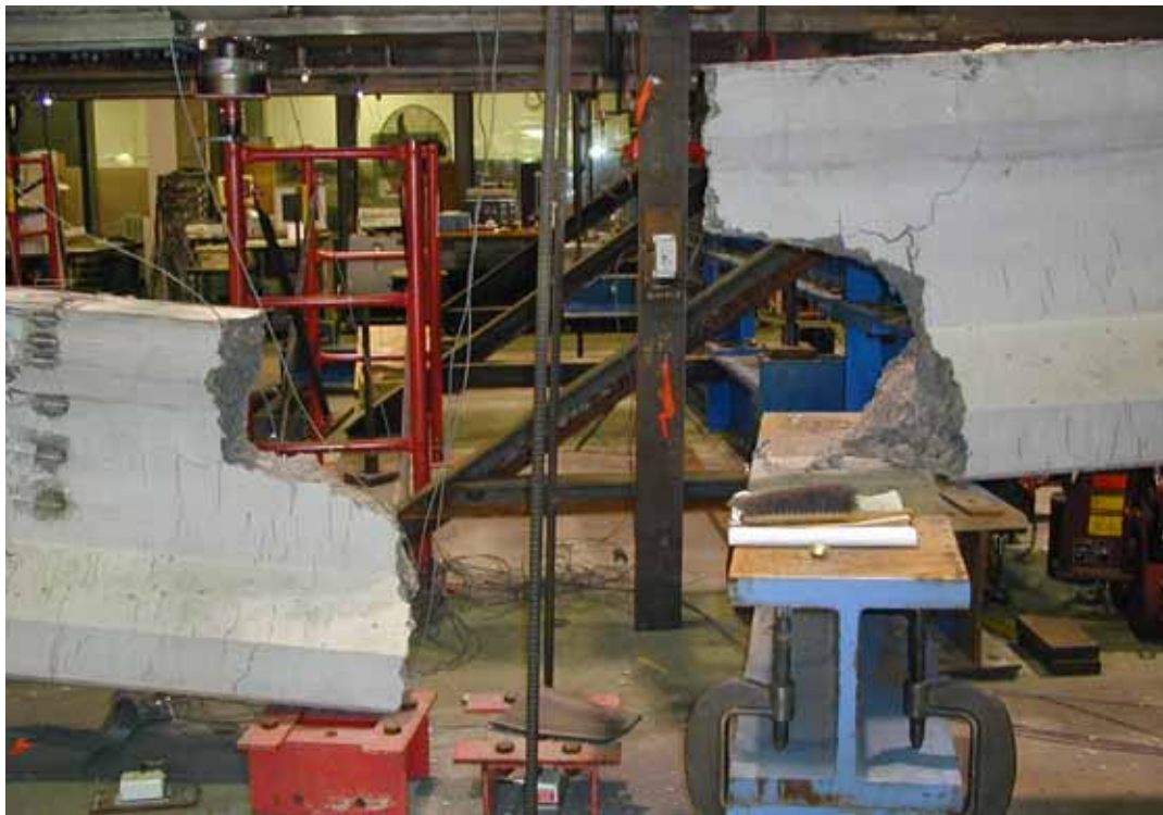
Figure 18. Photo. Girder 80F immediately after failure.
