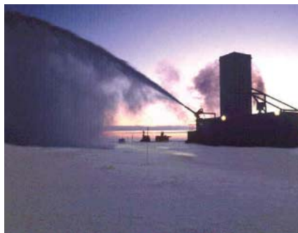
Tanker spraying water to build up ice surface.
