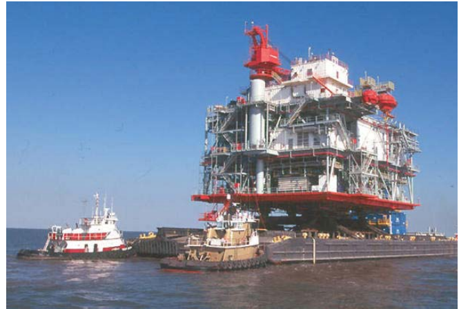
Above: The deck quarters of Petronius being transported offshore. Left: Petronius structure. Photos courtesy of Chevron.
