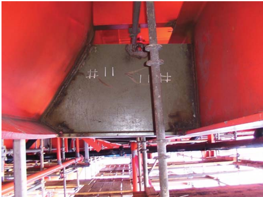
Left: Picture of Petronius repair before painting was completed. Below: A view of Petronius ' damaged deck plate girders. Photos courtesy of Chevron.
