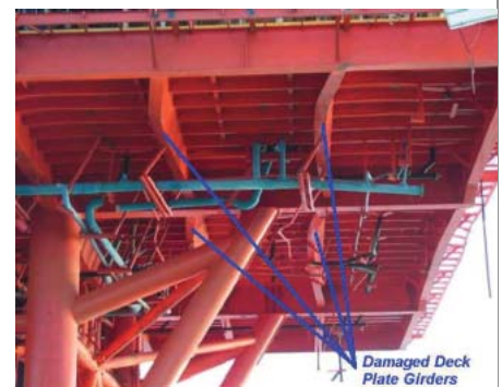
Left: Picture of Petronius repair before painting was completed. Below: A view of Petronius ' damaged deck plate girders. Photos courtesy of Chevron.
