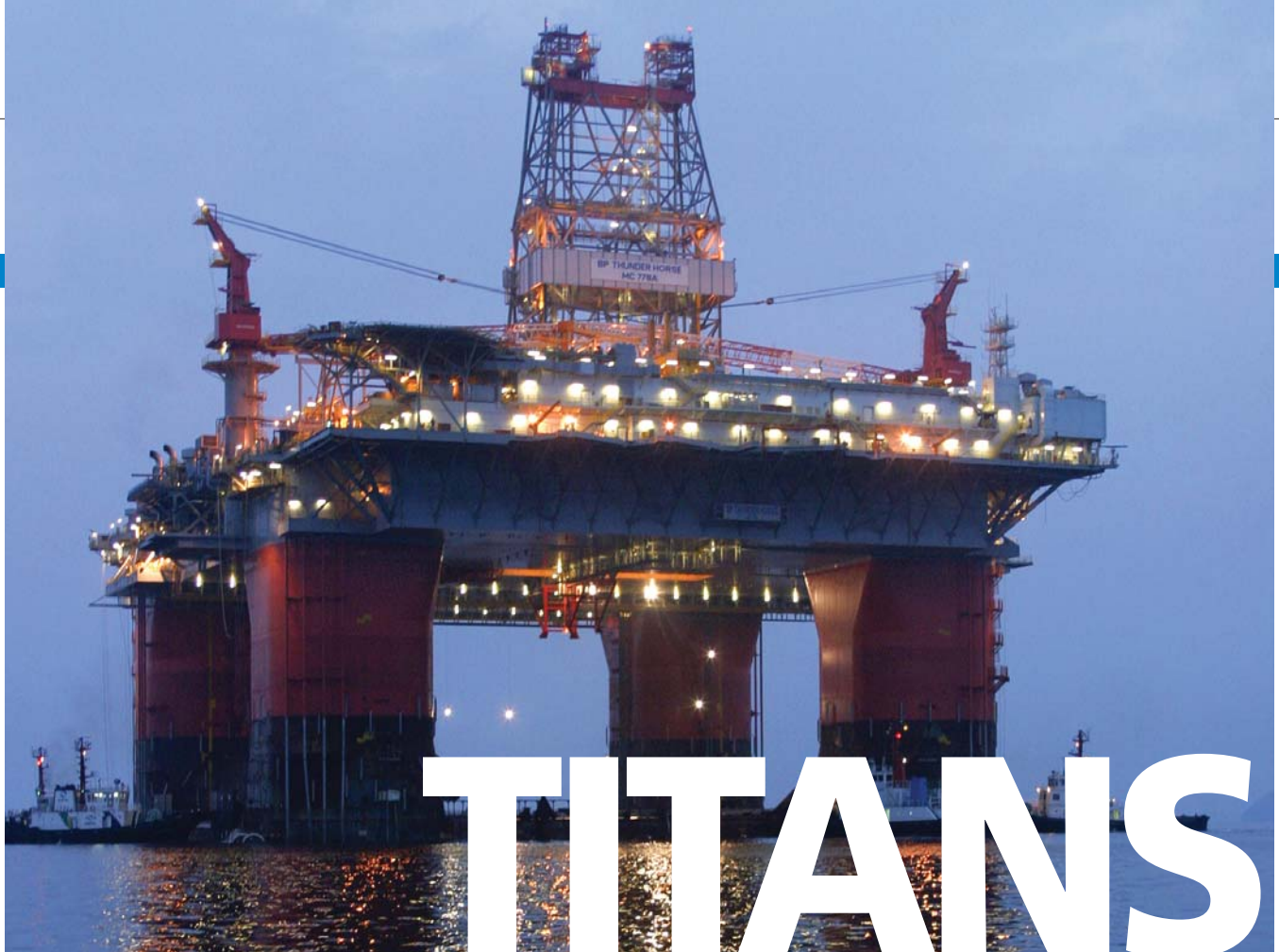
Thunder Horse facility at night. Photo courtesy of BP Exploration & Production.
