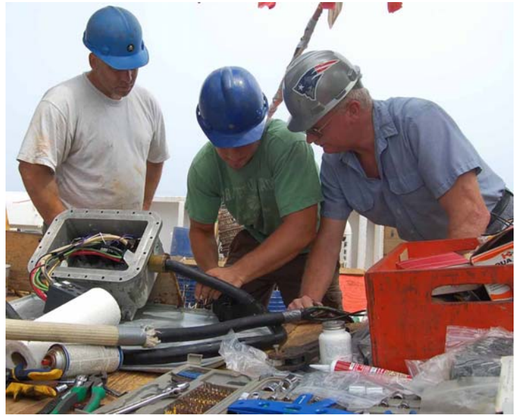
Chief Scientist Vic Nordahl, Chief Boatswain Jon Forgione and Chief Engineer Patrick Murphy discussing the best way to reattach the pump power cable to the dredge.
