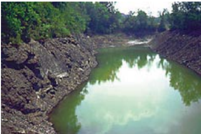
Prior to reclamation this abandoned coal mine contained dangerous highwalls, hazardous water bodies, and spoil material. The mining ended in 1952. Photo: Chuck Meyers, Office of Surface Mining.
