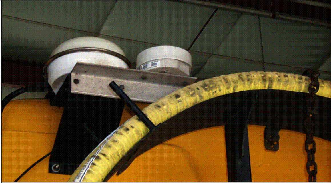
Figure E-3. Onvoy Antenna (right) shown next to QUALCOMM antenna (left)
