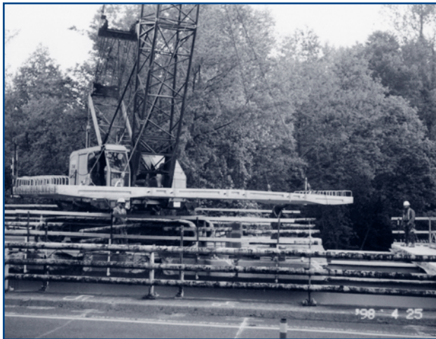
Full-depth deck panels for the George Washington Parkway in McLean, VA
