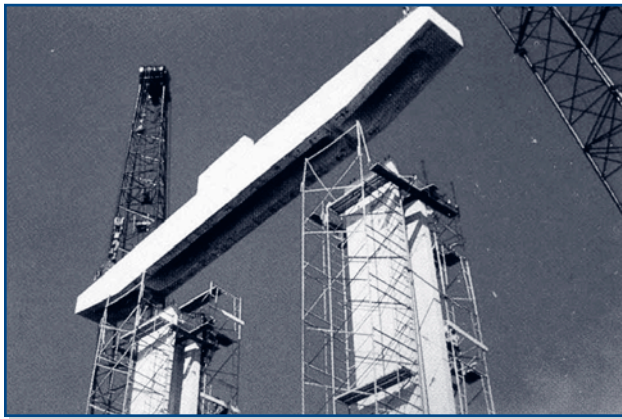
Prefabricated superstructure caps and columns
