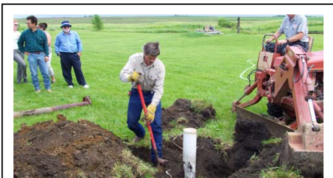
Well Sealing Demonstration hosted by many SWCDs throughout the state.
