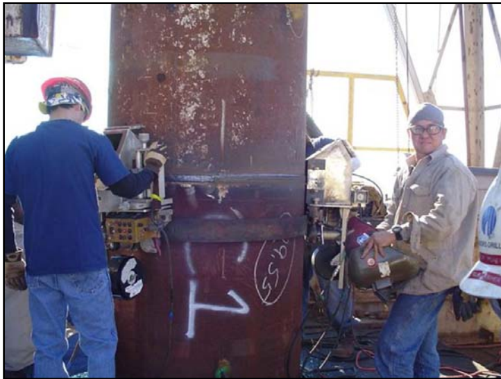
Figure 8: “UT”ing the welds, 48-in drive pipe
