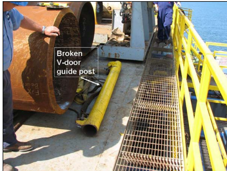
Figure 7: Broken right side V-door guide post
