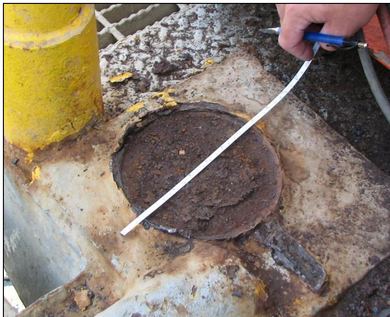
Figure 16: Location, welded base of V-door guide post to rig floor
