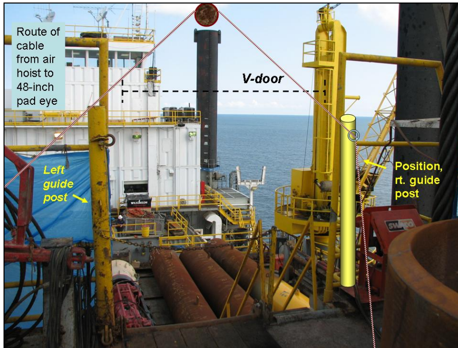
Figure 10: Rig-up method to attempt to rotate 48-in drive pipe
