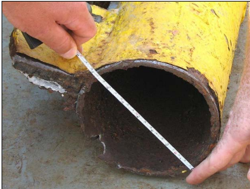
Figure 15: Base, broken right side V-door guide post
