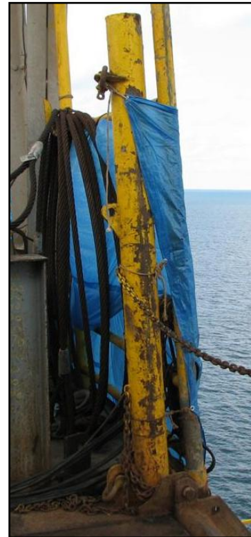
Figure 13: Left V-door guide post
