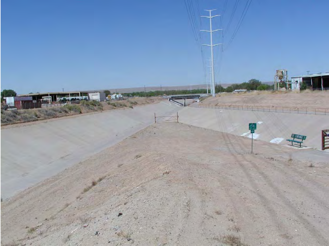
South Diversion Channel at the Tijeras Arroyo (Lower South Diversion)
