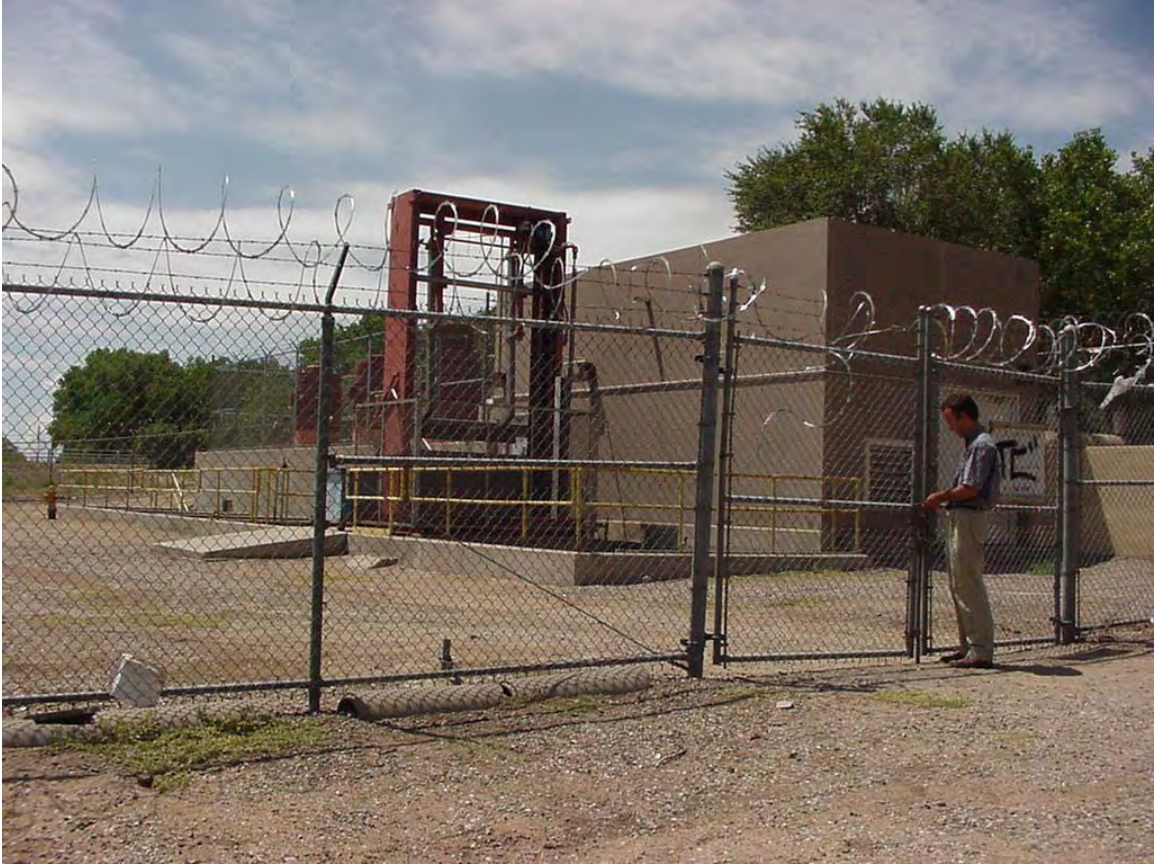
Barelas Pump Station
