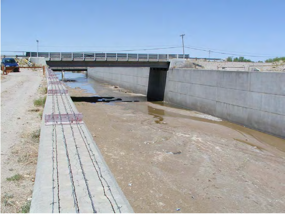
North Diversion Channel at Edith (North Diversion – Edith)
