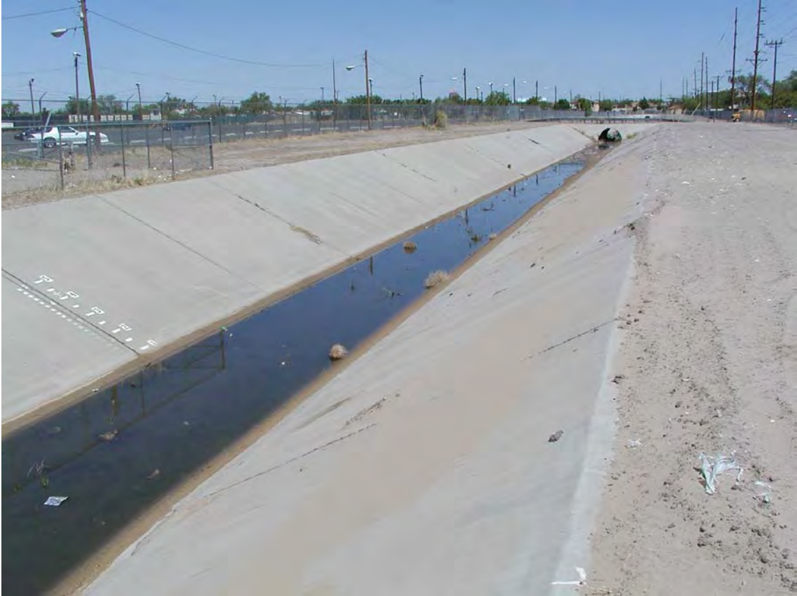
San Jose Drain at Woodward (San Jose)
