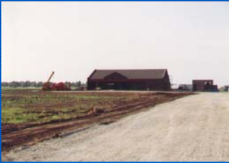
Office construction, June 1994
