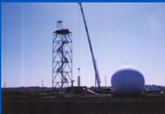
Construction of Doppler radar, April 1995
