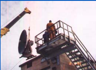
Installation of upper-air observing equipment, February 1995
