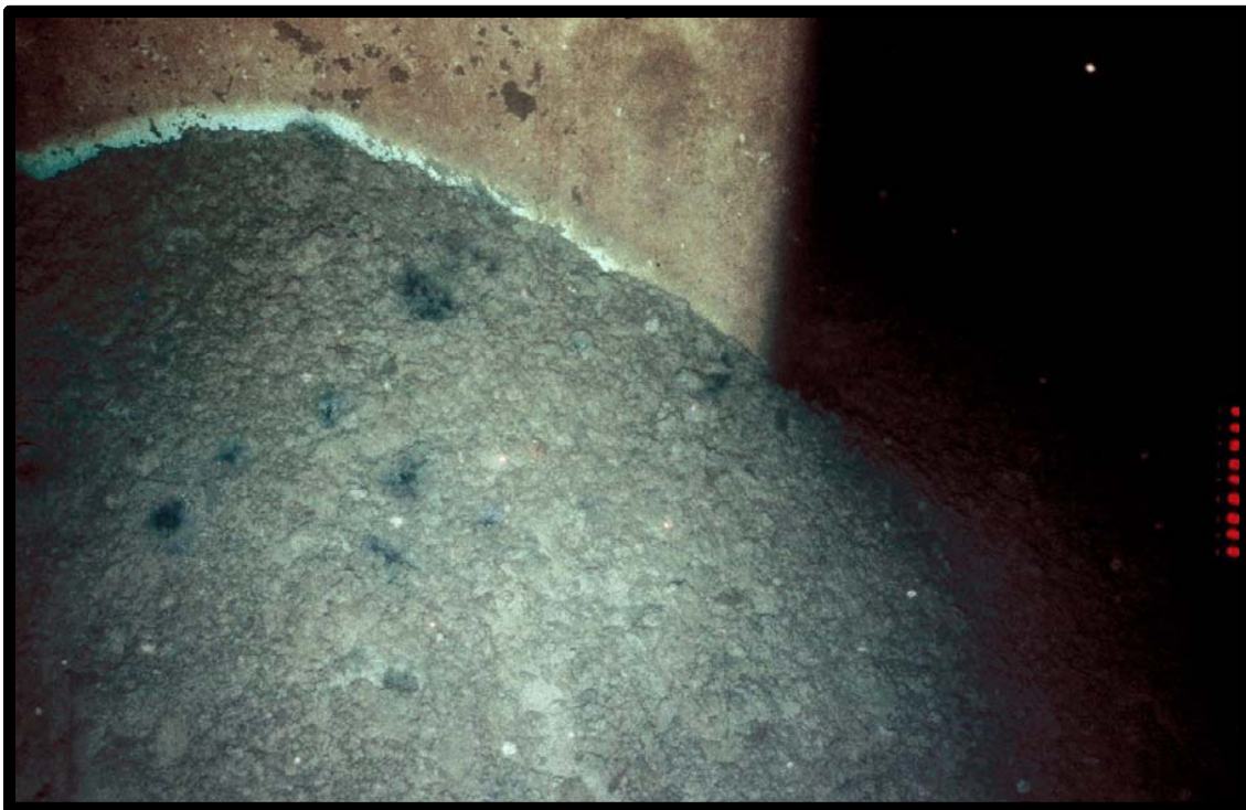
Photo 4 - Muds and cuttings accumulation near the base of a Ewing Bank Area Block 305 platform leg. The vertical relief of the accumulation was approximately 0.3 to 0.6 m (1 to 2 ft).
