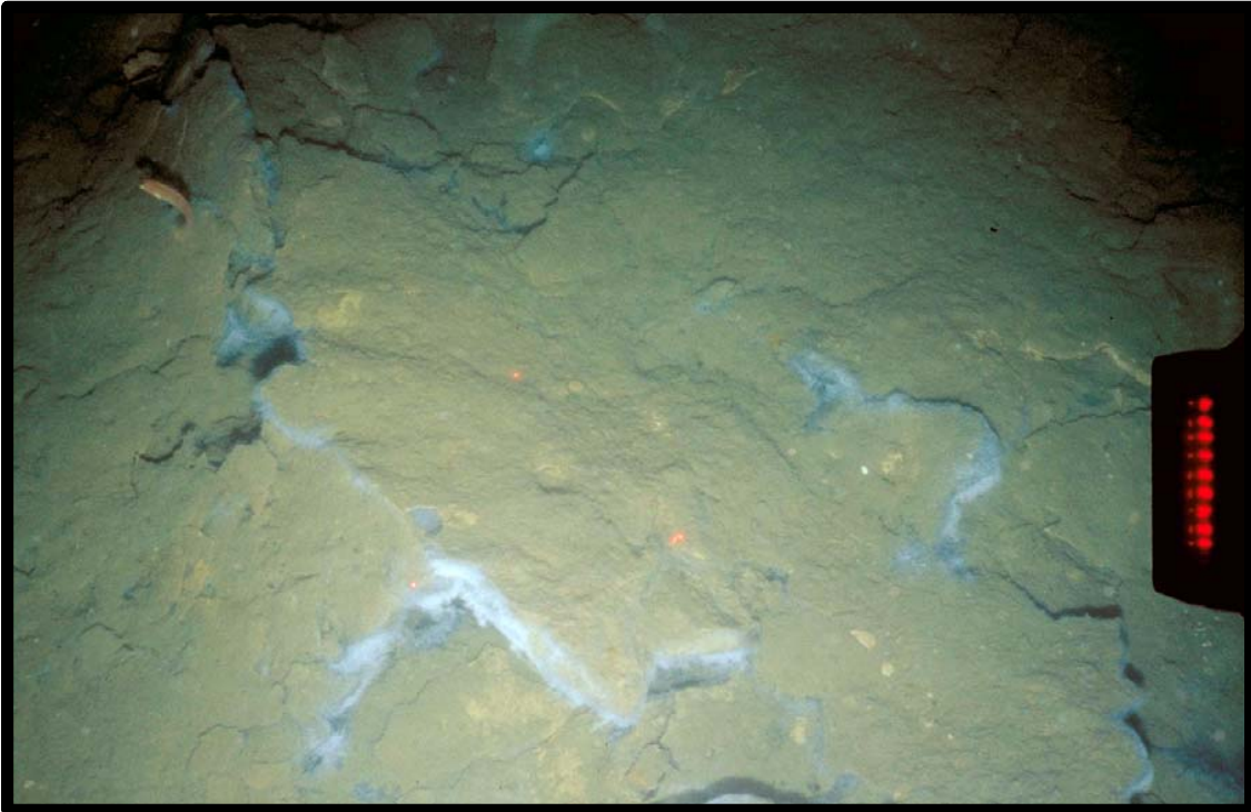
Photo 15 - A fractured veneer of concrete grout overlying sediment in close proximity to the Eugene Island Area Block 390 wellhead structure. A surficial layer of white filamentous material (? Beggiatoa sp.) is visible along the fracture lines.
