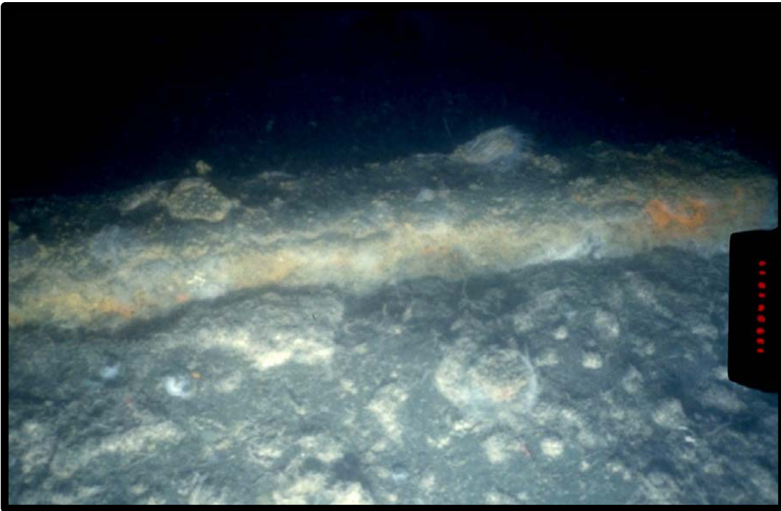
Photo 21 - Sacrificial anode partially buried by accumulation of suspected discharges along the northeast base of the Main Pass Area Block 288 platform. White filamentous mat (? Beggiatoa sp.) is visible overlaying portions of the darker sediment.
