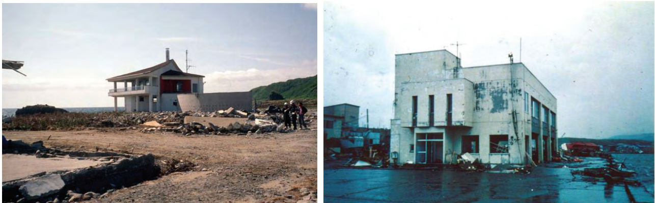
Figure 2-13 Examples of reinforced concrete structures that survived the 1993 Okushiri Tsunami: vista house at Cape Inaho (left); and fish market in Aonae (right) (Photo courtesy N. Shuto).
