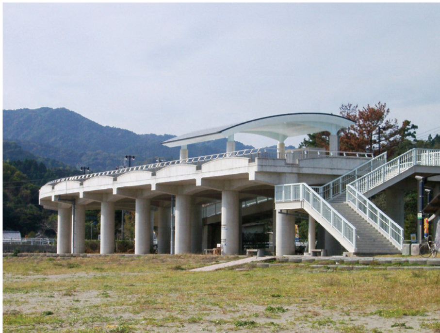
Figure A-3 Refuge at Shirahama Beach Resort (Photo courtesy of N. Shuto).
