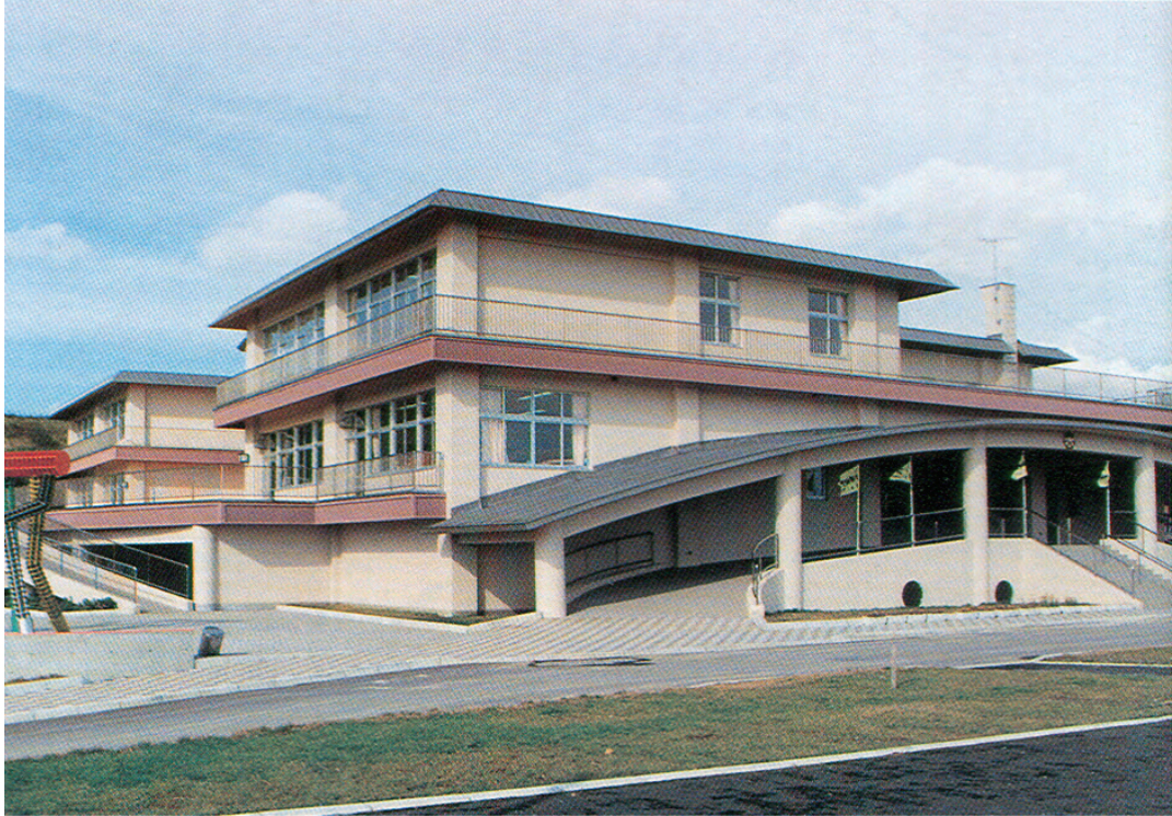
Figure A-6 Aonae Elementary School. Upper floors are intended for use as tsunami refuge space.
